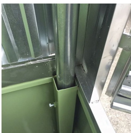
Tubulars for fixing in the basin
