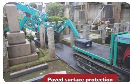
Paved surface protection
