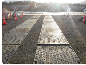
Roadways for heavy trucks
