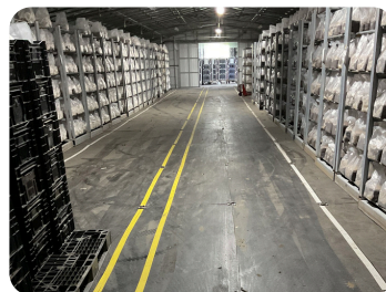
Temporary flooring in warehouse
