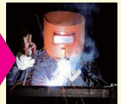
Resume welding works.
